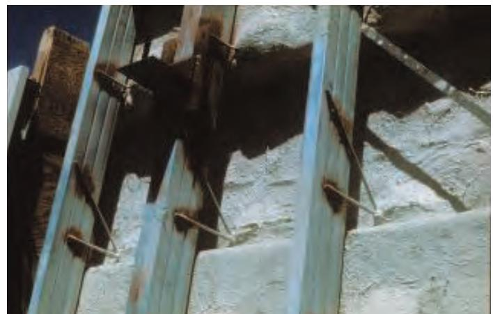
Figure 23 - Truss anchors with galvanized 6-inch studs
