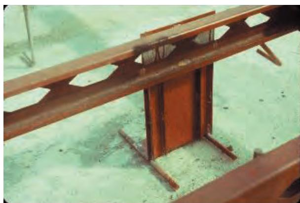
Figure 24 - Bar gravity anchor
