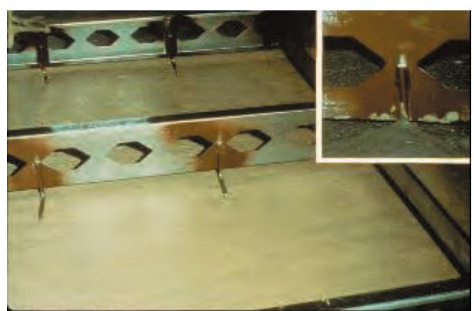
Figure 25 - Galvanized steel studs and stainless steel anchors
