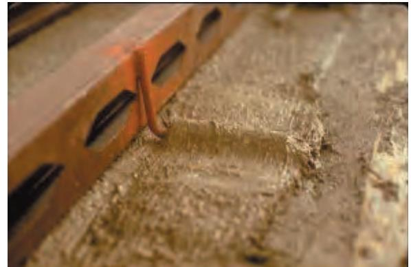
Figure 12 - Anchor and bonding pad
