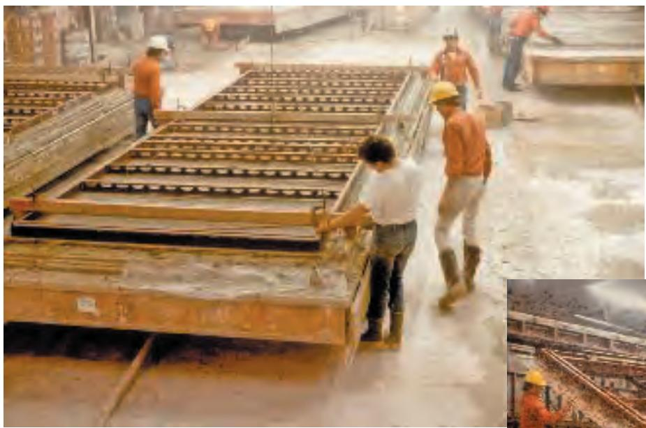
Figure 10 - Positioning (above) and stripping (right)
