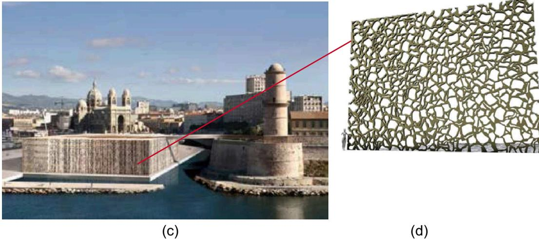
**Figure 1:** Examples of architectural applications in Ductal<sup>®</sup>: a) thin-shelled canopies at Shawnessy LRT station in Calgary (2004); b) perforated façade panels in the ZAC apartment building in Paris; c) perforated roof and envelope of the future Jean Bouin Stadium near Paris (model, Ref. [2]); d) perforated façade panels and footbridge at the MuCEM in Marseille.
