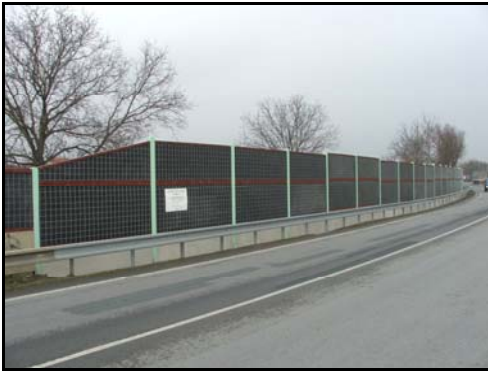
Figure 6: Implementation of absorptive wall
