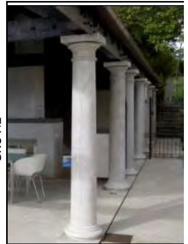
Figure 20: Decorative Columns, Auckland, NZ
