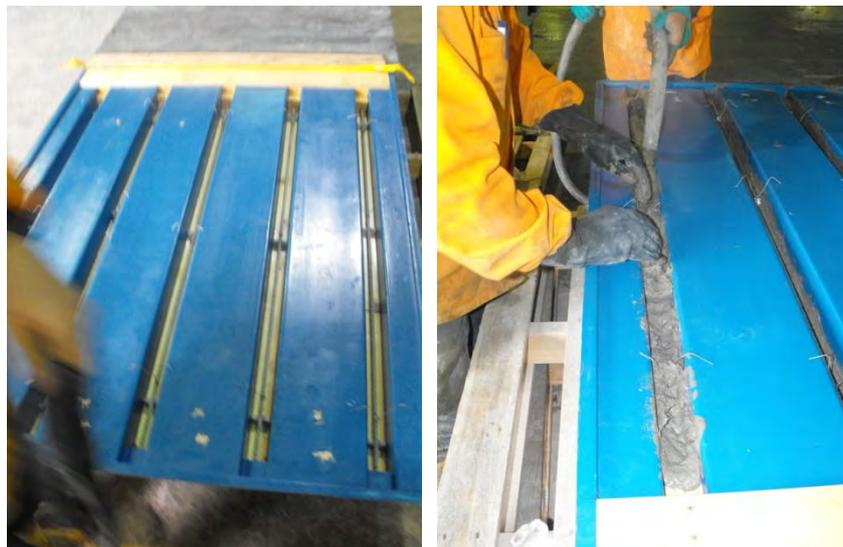
Figure 10 Formwork mould, FRP bar position and unit casting
