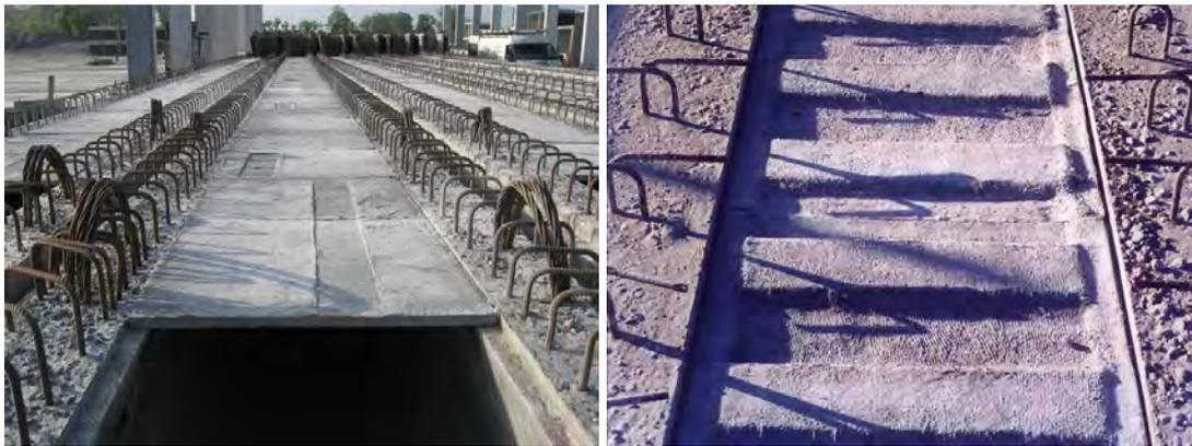
Figure 8 GRC permanent formwork (left: flat (Shay Murtagh); right: single corrugated (BCM GRC))
