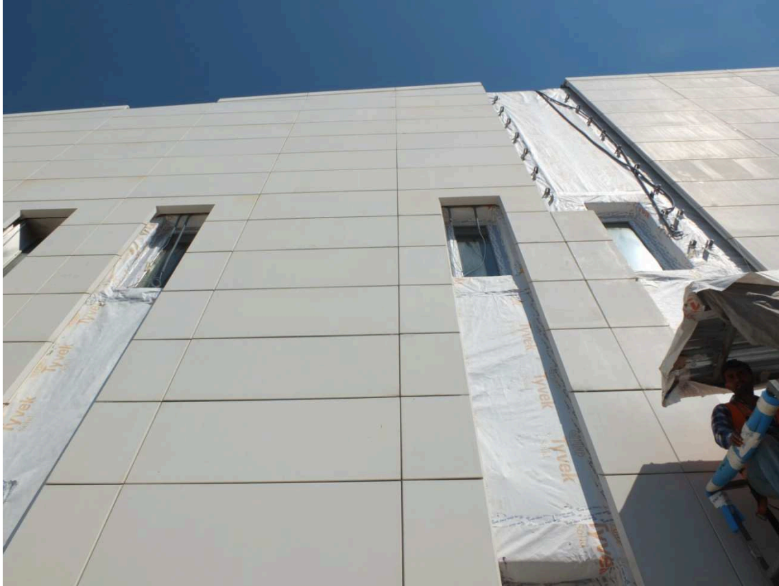
Figure 1. Façade of the Tüpraş RUB
