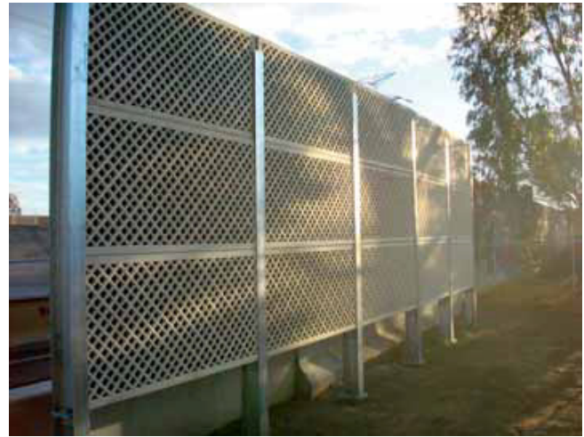
Figure 6: GRC absorption panels, Australia.
