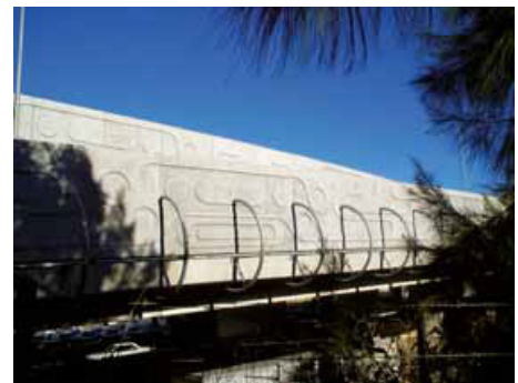
Figure 3: Glebe Island off-ramp, Australia – GRC reflective barriers.
