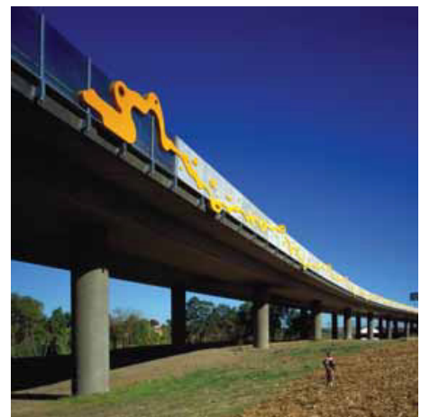
Figure 4: M4 motorway, Parramatta, Australia – GRC and acrylic panels.
