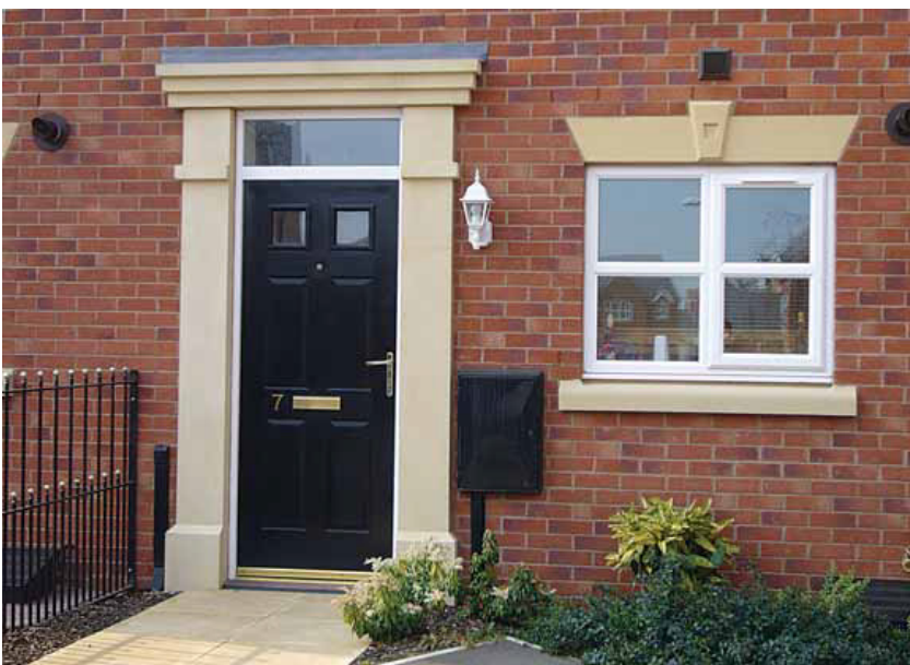
Figure 3: GRC door surround creates a dramatic entrance.
